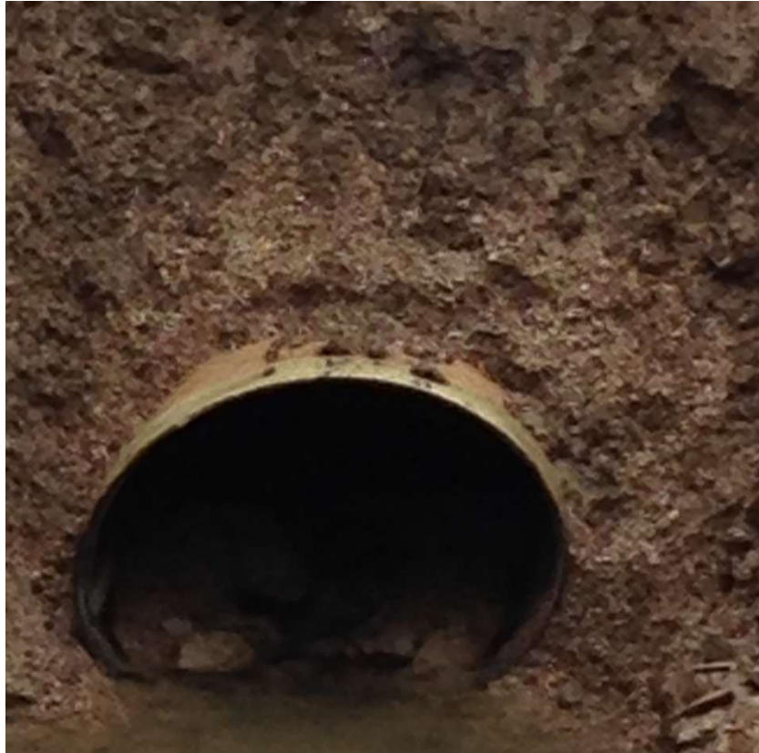
Figure 6: Photographs of Various Installations Where Finer Soil has Migrated into Coarse Soil
